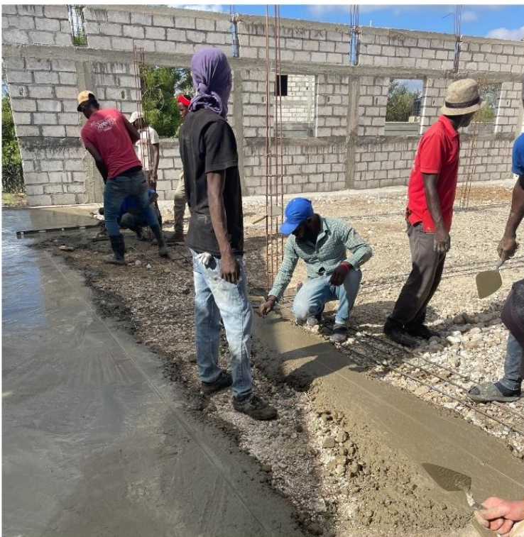
Laying a concrete floor for the church.
