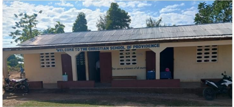
Classrooms of the Christian School of Providence.
